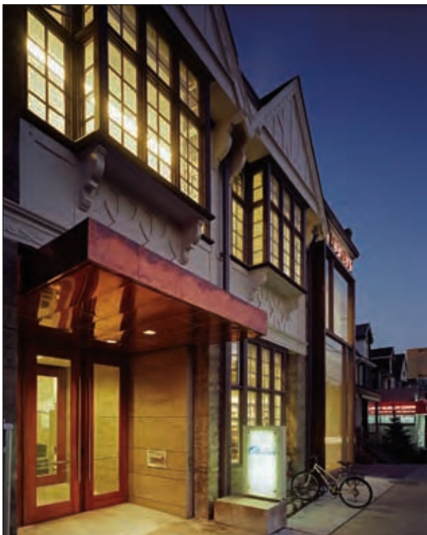
Façade restored: Using materials characteristic of Pape's original entrance, the restored façade features a copper canopy over a teak front door and improved presentation of the original bay windows on both levels.
