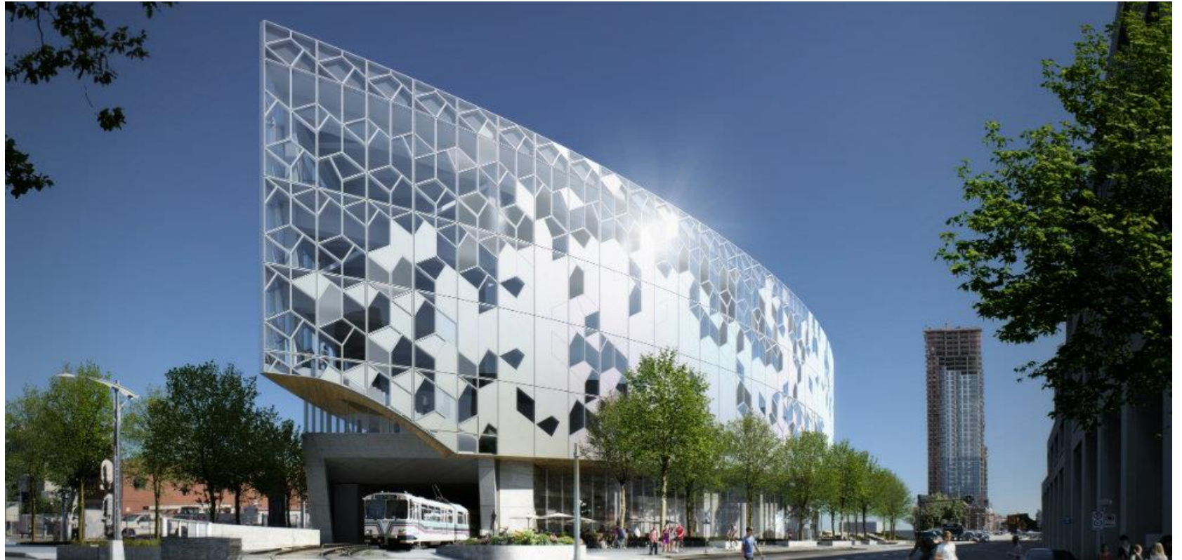
Fig. 2. Calgary Central Public Library from: https://calgarylibrary.ca/central-library/room-bookings/
