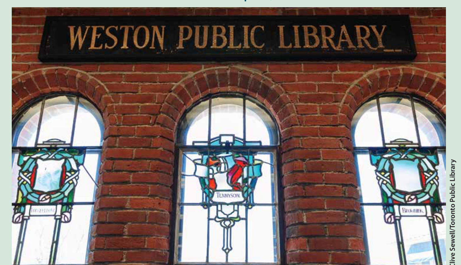
Stained glass windows, west wall, facing Weston Road, 2014
