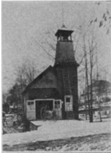
East Toronto Fire Hall No. 1, Spruce Hill
